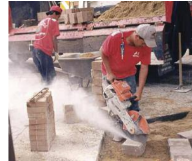
Dry sawing concrete
