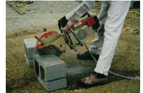
Wet sawing concrete Water is added at saw blade
